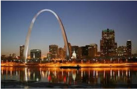
Fig.3.1.1. Gateway arch. in St. Louis, USA
