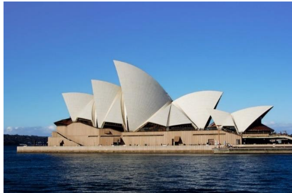
Fig.7.2.1. The Sydney Opera House is likened to sea shellfish and ship sails. https://www.boredart.com/2015/04/the-art-of-architecture-and-the-beauty-of-it.html
