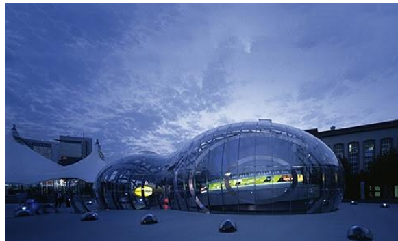
Fig. 1. Blob form of BMW Bubble Pavilion in Germany https://archello.com/project/bubble
