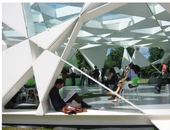
Fig.6.1. The structure created by rotating and copying the basic geometric object (square) and its subsequent application to the pavilion object, also represents its construction, Serpentine gallery pavilion, London, design: Toyo Ito
